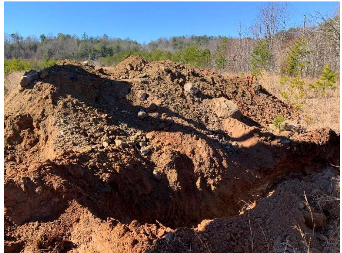
View of Test Pit Excavation
