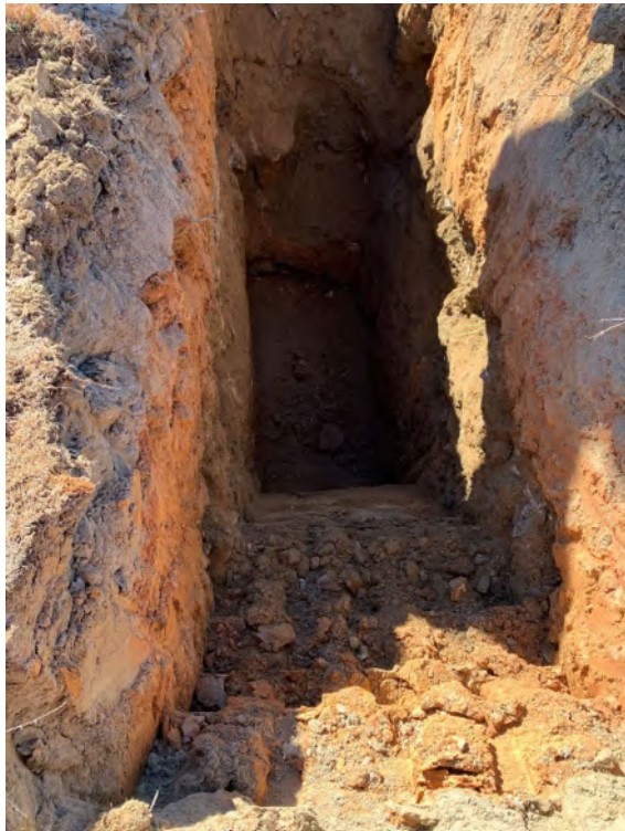
View of Excavated Material
