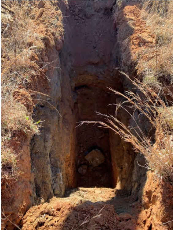
View of Excavated Material
