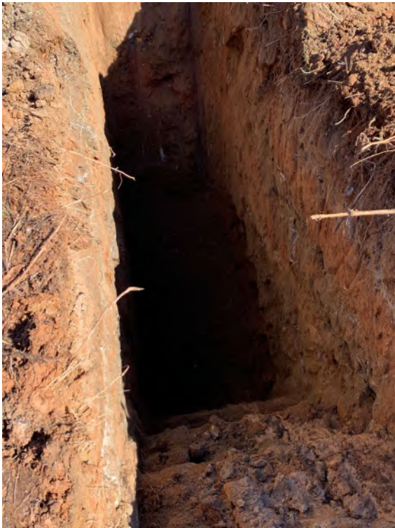
View of Excavated Material
