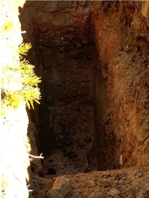
View of Excavated Material
